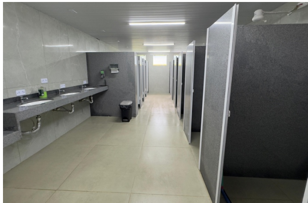
Remodeled Girls' Bathroom at ARCA
